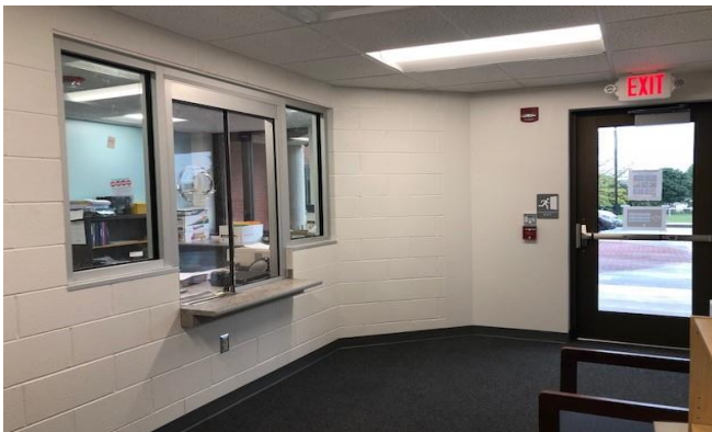
New Secure Entrance at the Elementary School
